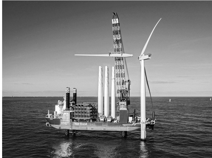
Gemini offshore wind farm, under construction
