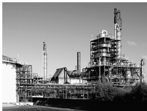
Chemical site Delfzijl: green chemicals production
