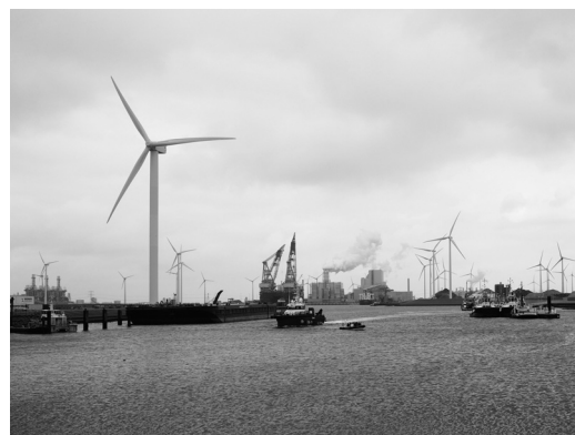
Port of Eemshaven: the Energy port
