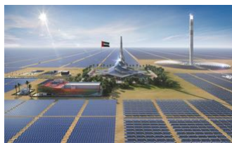
Mohammed Bin Rashid Al Maktoum Solar Farm Dubai; 3.000 MW ready, expansion to 5.000 MW
